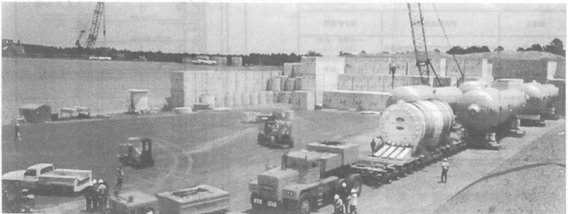
Photo 3 (Yankee Rowe) Unloading Work of Reactor Pressure Vessel Package at Barnwell, SC for Disposal
