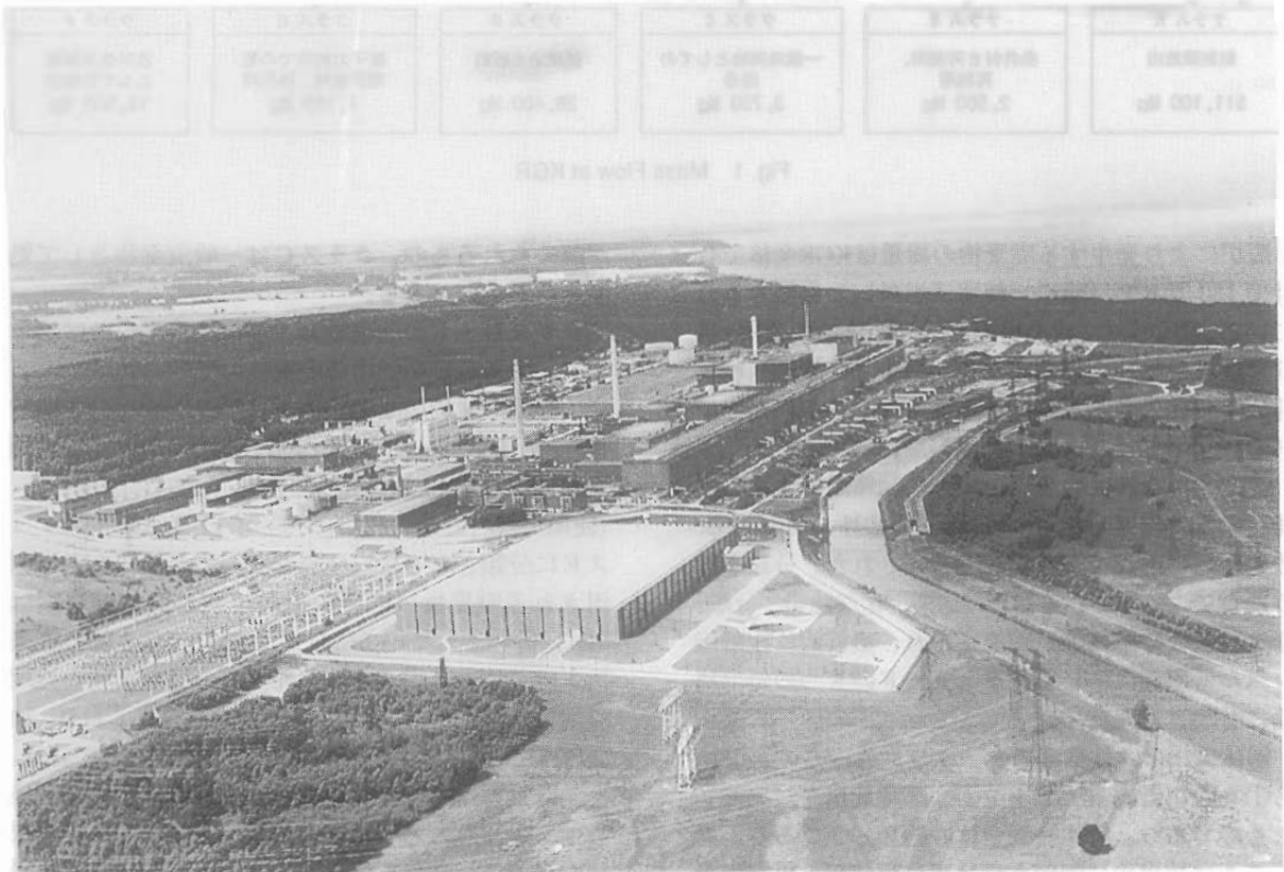
Photo 1 Overall view of Greifswald NPP site
