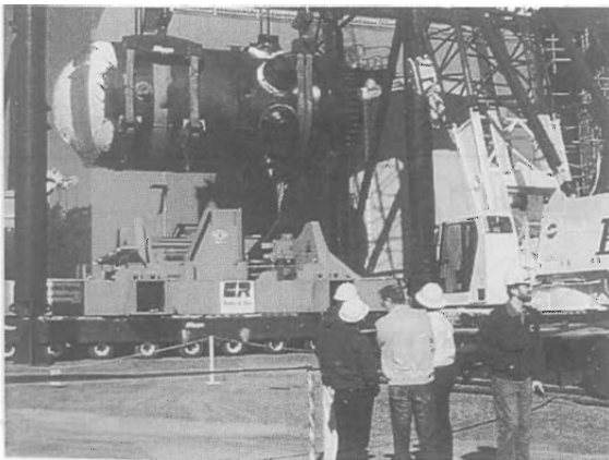
Photo 4 (Trojan) Loading Work of Reactor Pressure Vessel and Internal Package for Transport
